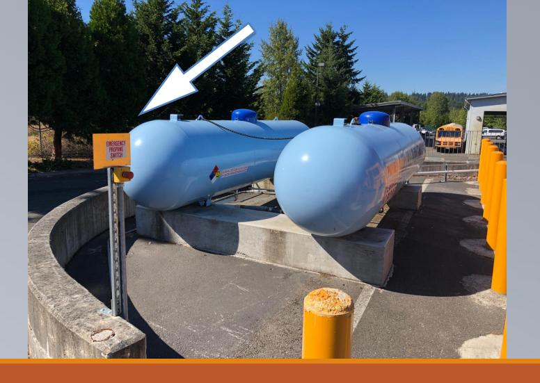
ALL emergency switches in the lot will turn off ALL fuel systems. Although this switch 'says' emergency propane switch...it will shut off all fuel systems - gasoline, diesel, propane and electric.
